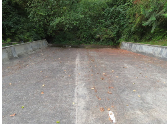
Dam Overflow Spillway
