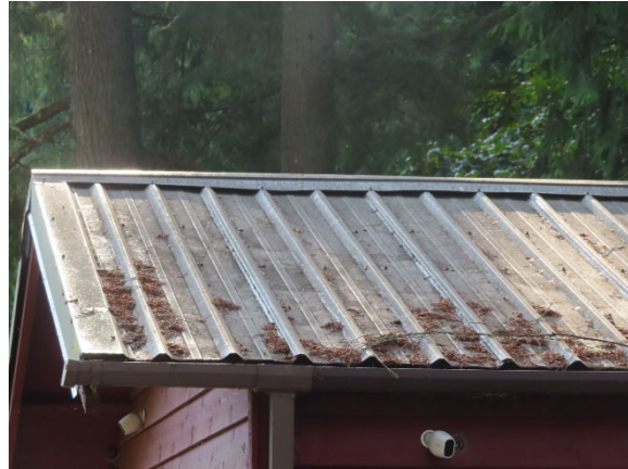
Roof of Office
