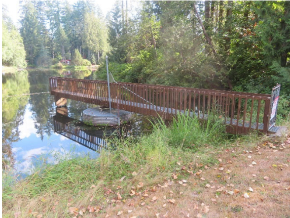
Bridge to Dam Outlet
